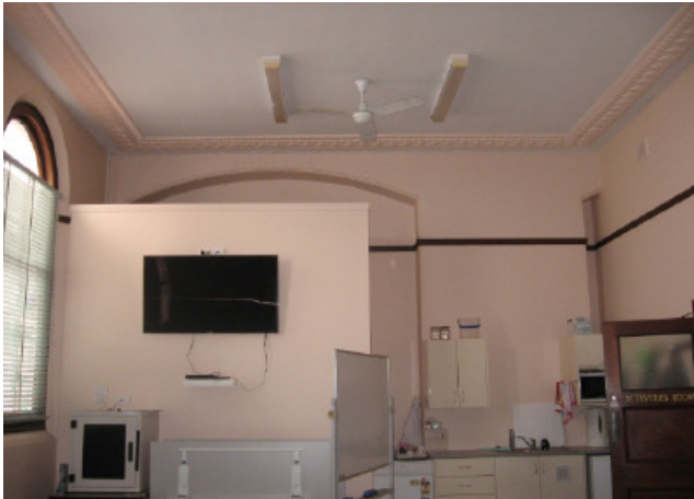
Figure 3.12 Looking west across one of the rooms created when the original council chamber was partitioned in 1936. The original chimney breast is visible behind the kitchenette (fireplace removed)
