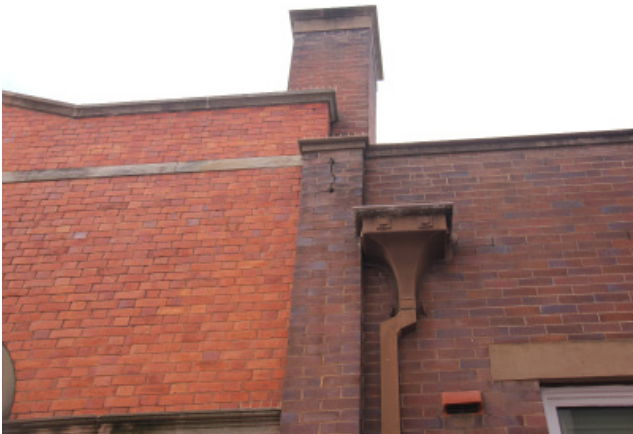
Figure 3.5 Brick pier and chimney of the southern elevation of the building indicating the junction between the 1887 building (red brick) and the 1936 addition (darker brown brick).
